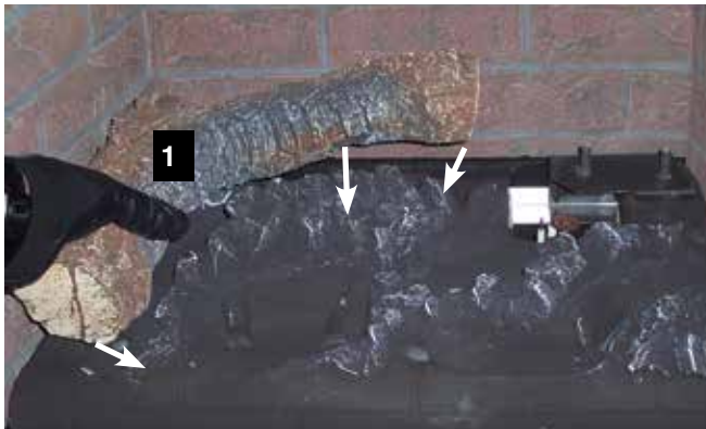
Log 1 location on burner
