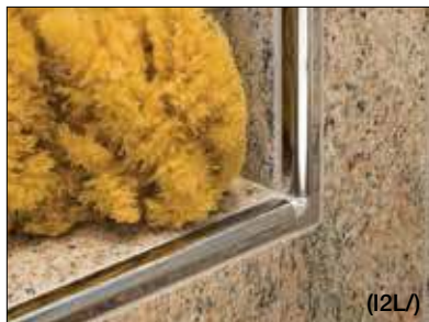
Sink corner with 3/8" (10 mm) radius (I2S/)
