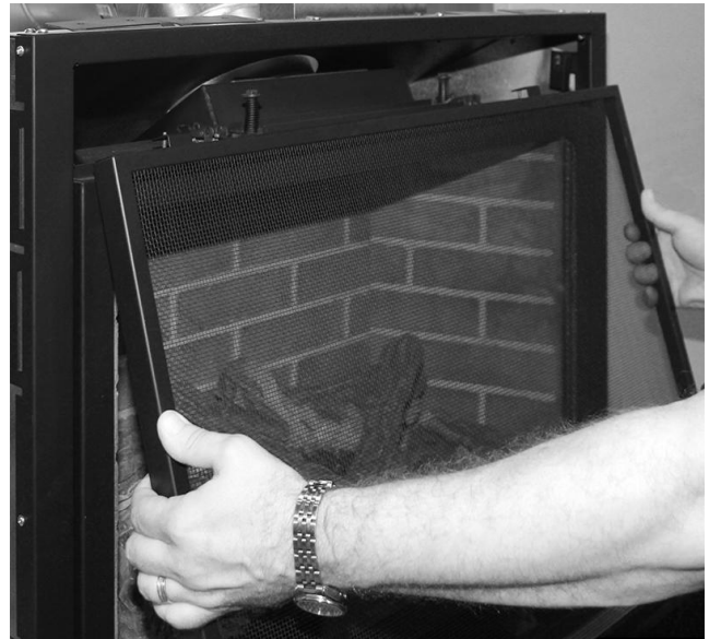
STEP 2: Locate the two small vertical studs on the firebox top. Slightly angle the screen upwards and line up the tab holes with the firebox studs.
